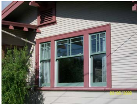
2" window recess from face of wall
