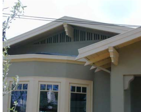
Vents as an architectural element
