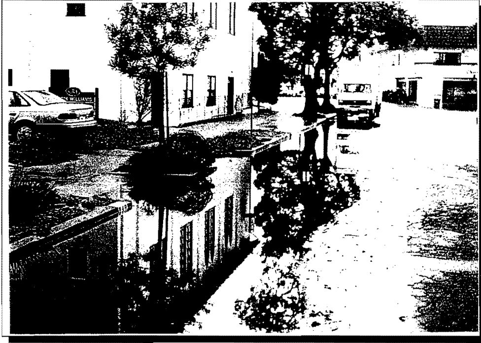
PONDING ON POMONA AVENUE NORTH OF SOLANO AVENUE JANUARY 1998
