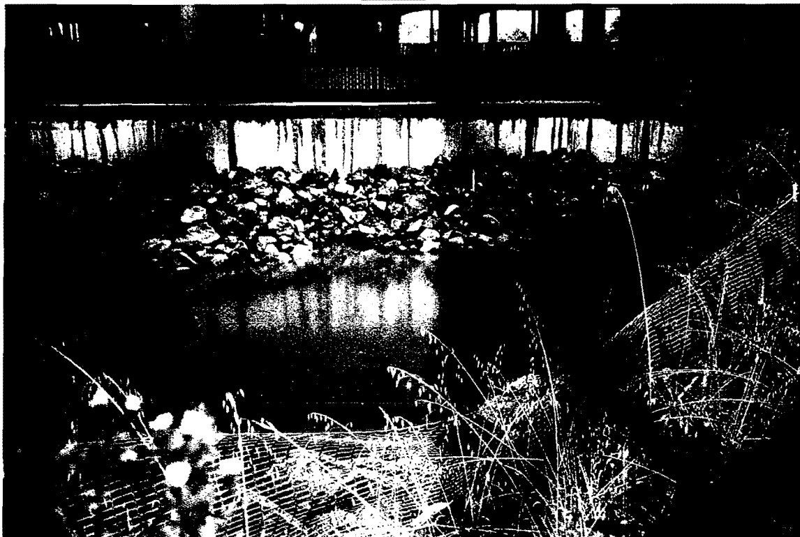
MARIN CREEK OUTFALL AT THE SAN FRANCISCO BAY MAY 1998
