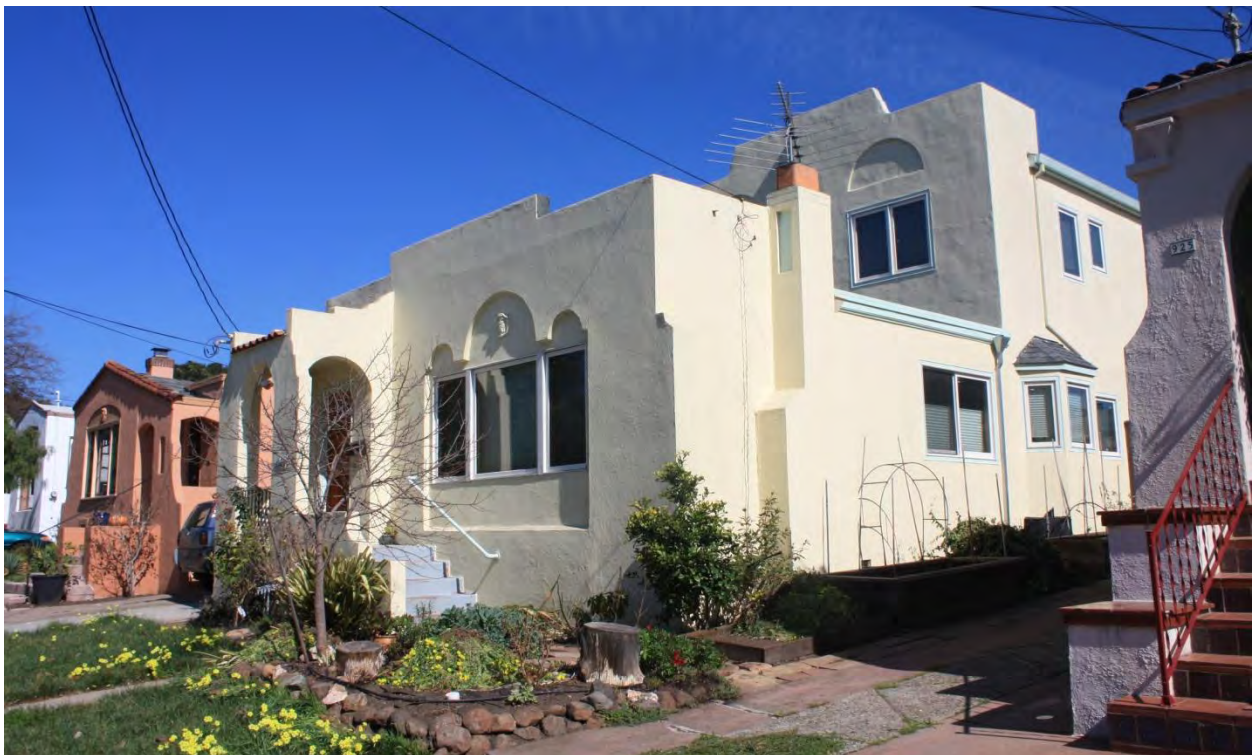
This second story addition incorporates many of the design features of the original home.
