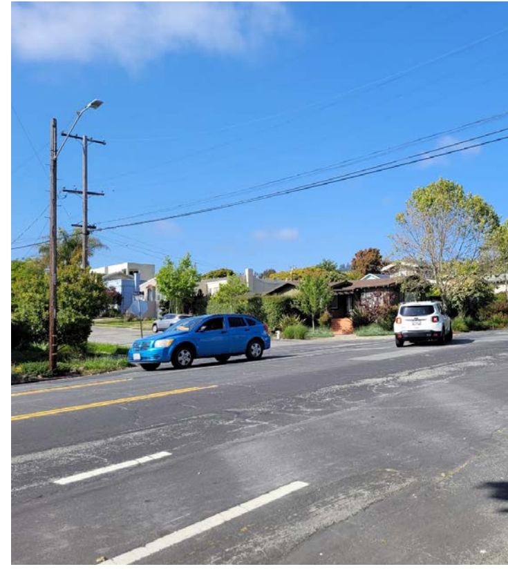
SITE PHOTO: DAY
