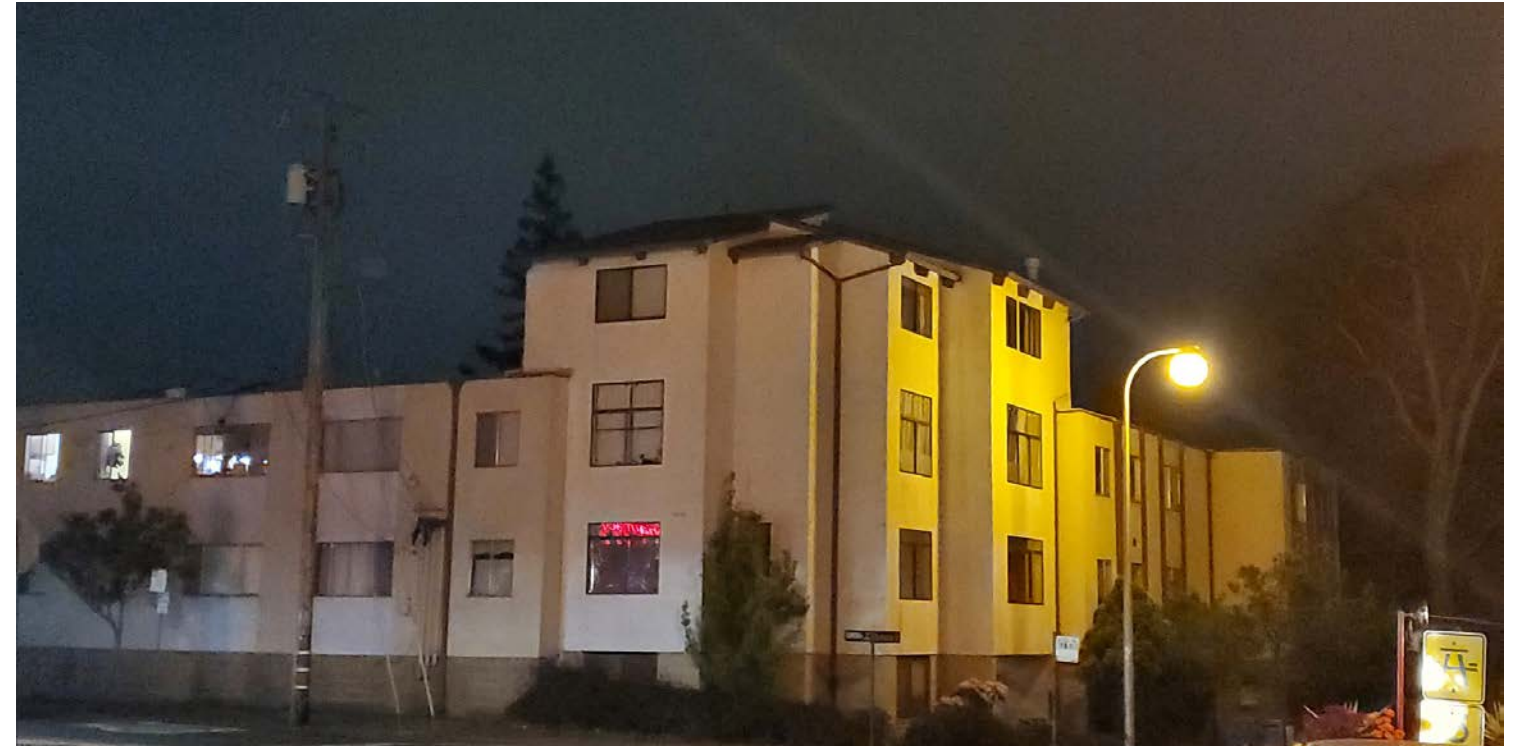
LIGHT TRESPASS FROM UNSHIELDED LUMINAIRE
