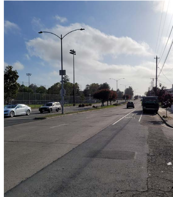
SITE PHOTO: DAY
