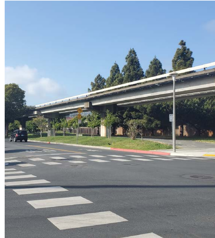
SITE PHOTO: DAY
