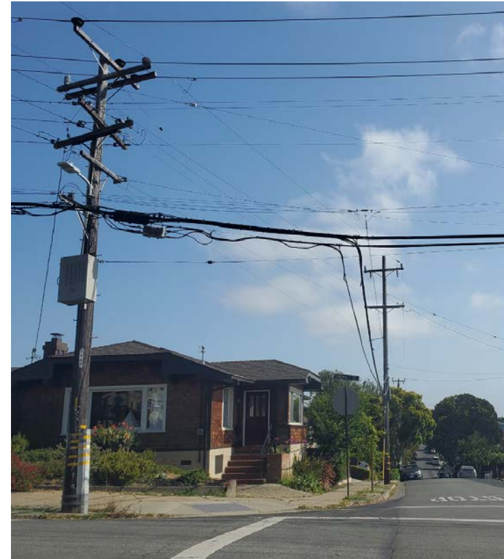
SITE PHOTO: DAY
