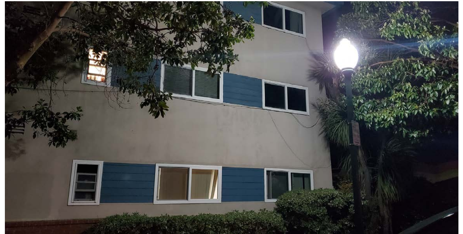
LIGHT TRESPASS FROM UNSHIELDED LUMINAIRE
