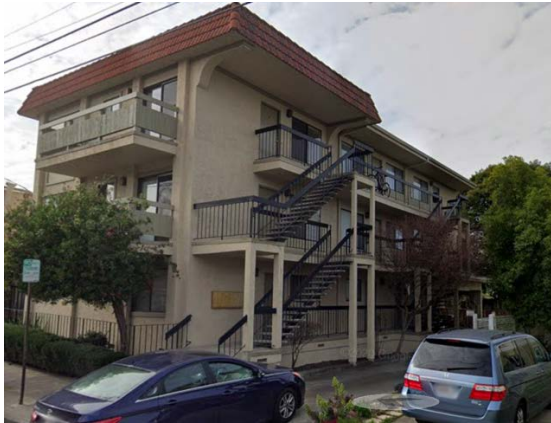
1a. 3-story, 8-unit. WFTS due to end bay parking at the rear (not visible)
