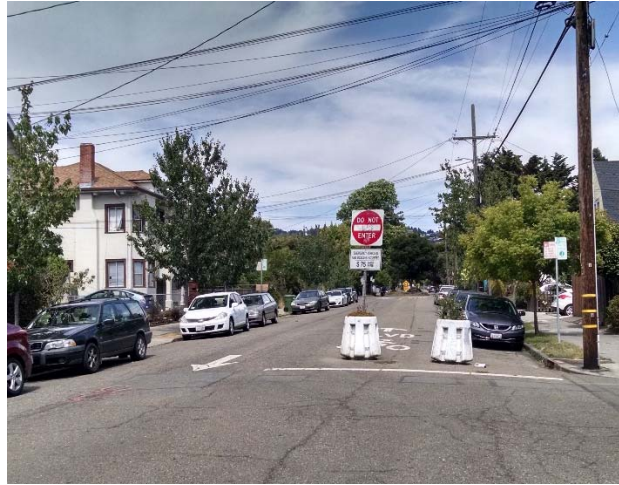
Figure 6 Partial Closure Example Russell Street, Berkeley, CA.
