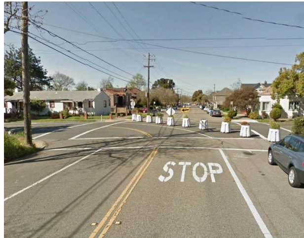
Figure 7 Traffic Diverter Example Berkeley, CA. Image: Google, 2017.
