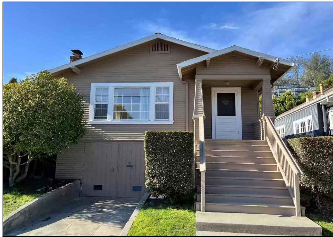
FRONT OF HOUSE (WEST)
