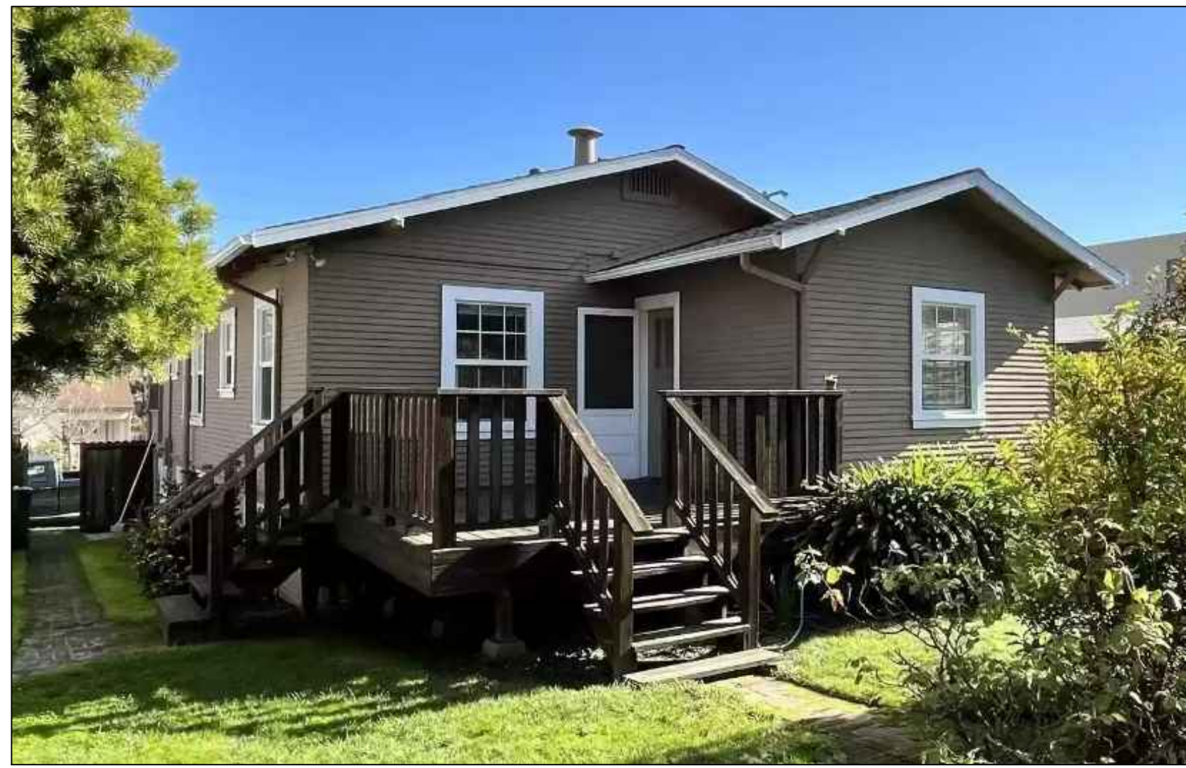
REAR OF HOUSE (EAST)
