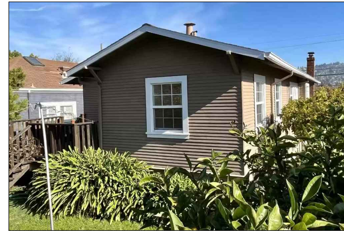
REAR OF HOUSE (EAST)
