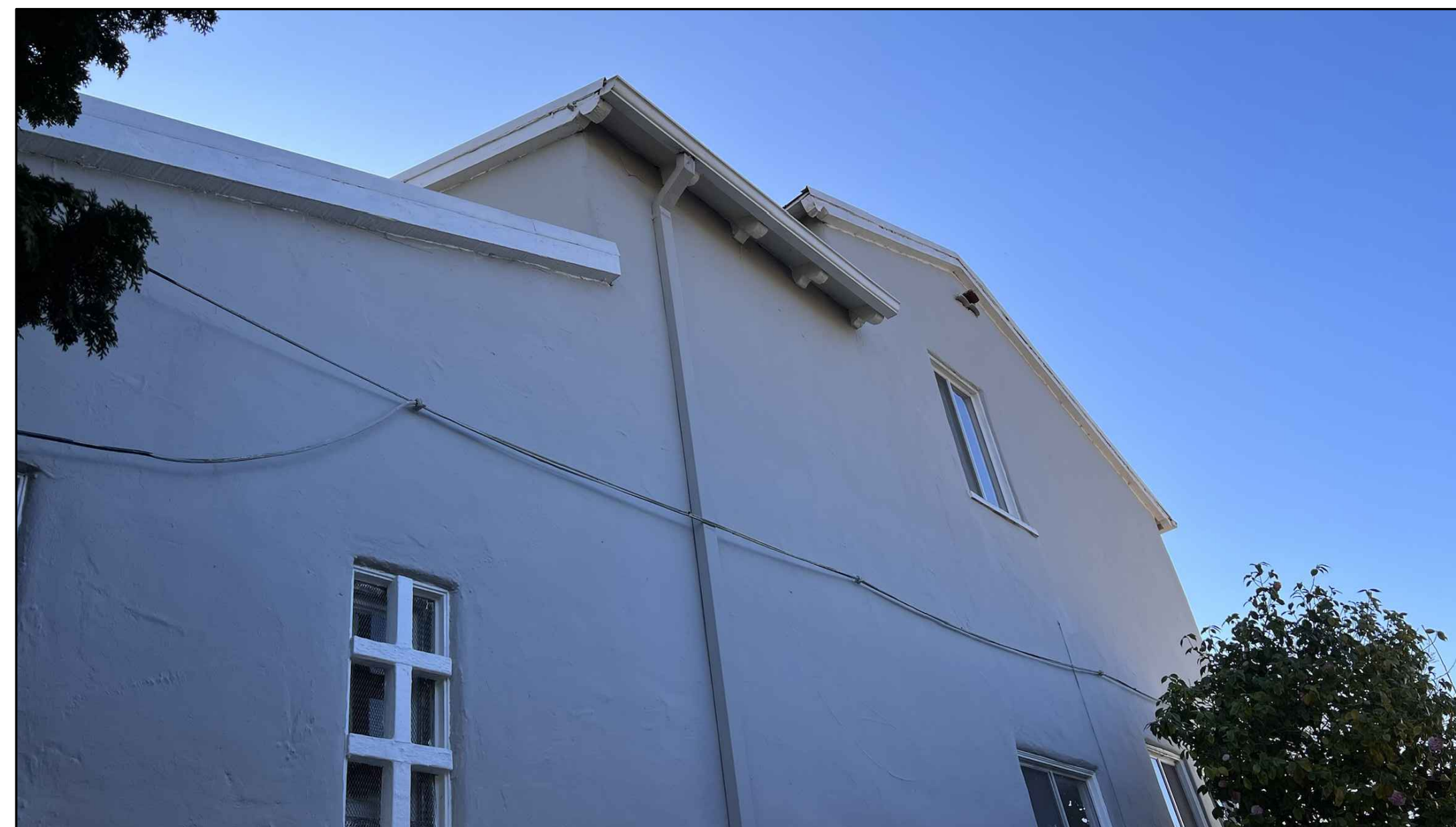
1020 ORDWAY - NORTH SIDE VIEW
