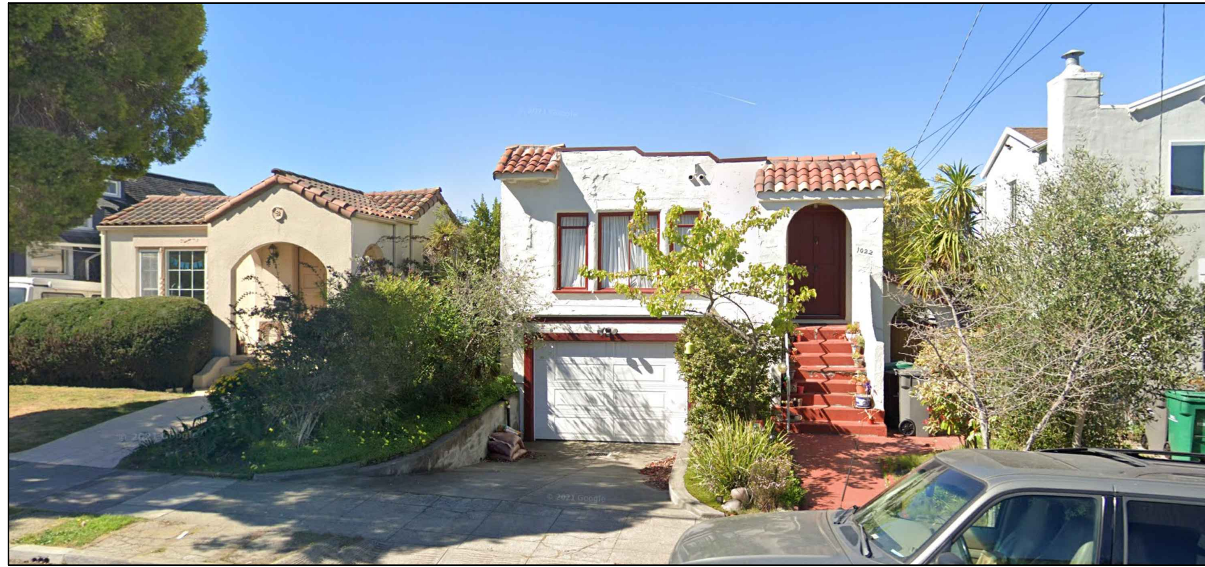
1022 ORDWAY - STREET VIEW
