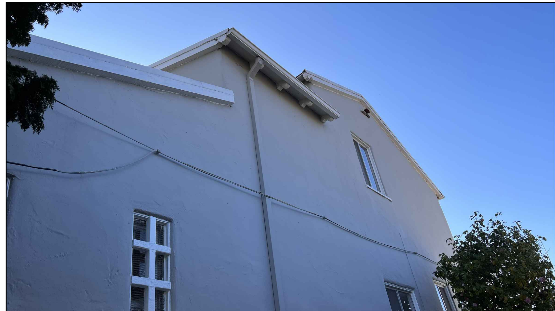
1020 ORDWAY - NORTH SIDE VIEW
