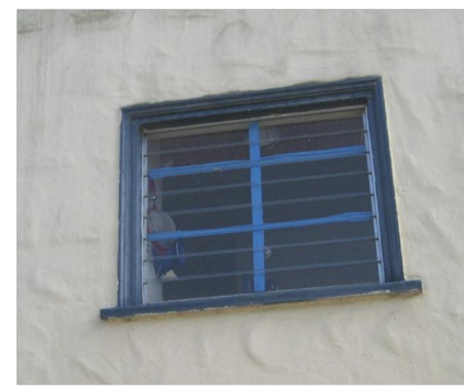
Sample digital exterior photo of window to be replaced
