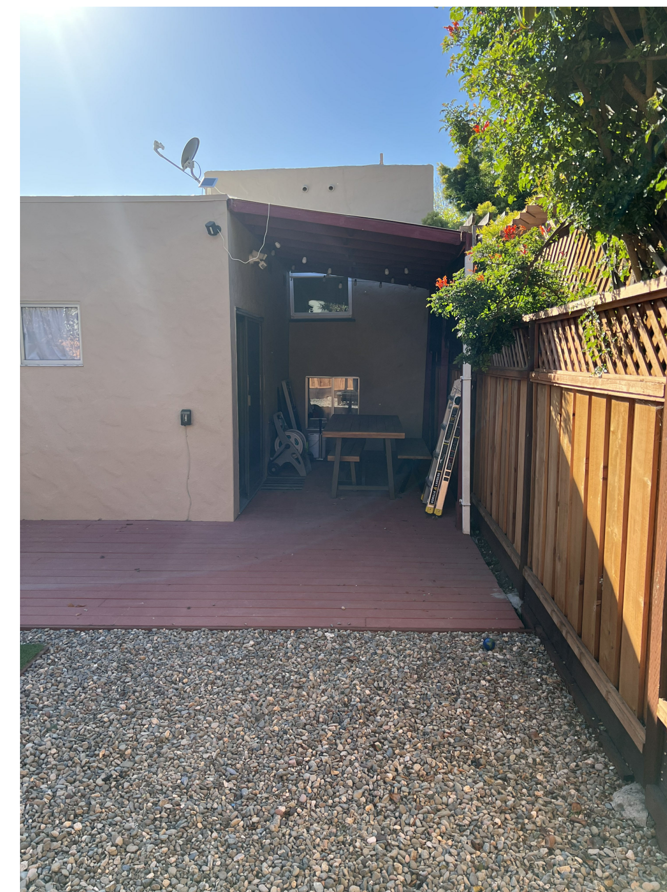
3 (E) COVERED PATIO PHOTO NOT TO SCALE
