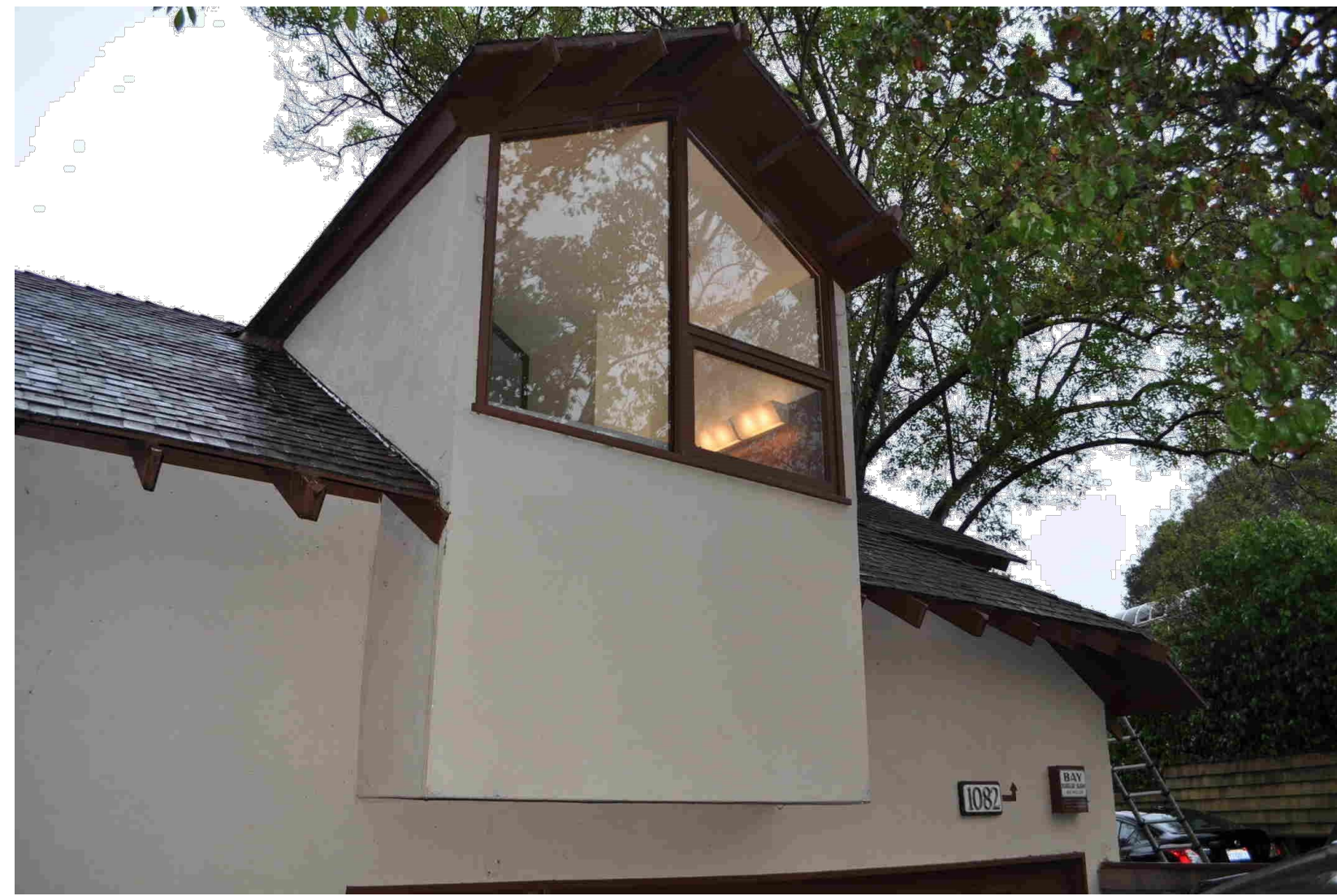
EAST WINDOW APPROACH
