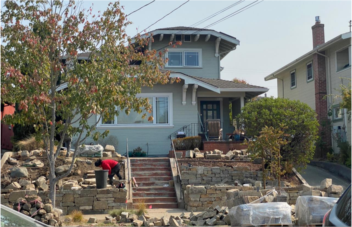
Image 3. New Stone Wall at 955 Ordway
