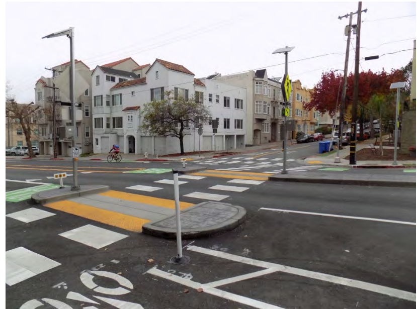
Figure 2.7. A Rectangular Rapid Flashing Beacon at an uncontrolled crosswalk in Berkeley that serves bicyclists and pedestrians.
