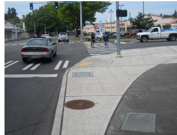
Figure 4.1. Example of the lifecycle of a curb extension: Short-term - temporary installation with paint. Medium-term - concrete repaving without moving the curb line. Long-term - permanent curb extension with shifted curb line.
