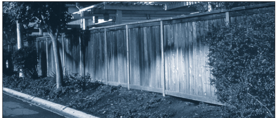
Damage to fencing from sprinkler irrigation.
