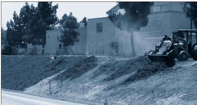
Shredded mulch is placed on miles of freeway hillsides by Caltrans.
