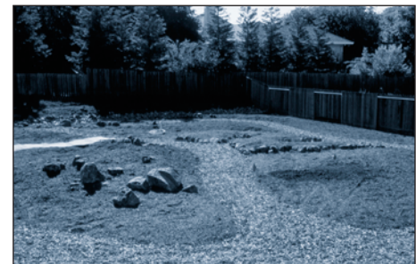
Sheet mulched site is ready for planting.
