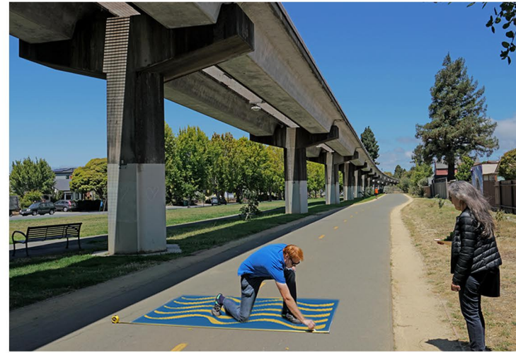
Embed artwork in asphalt at 3 locations - float in soft concrete
