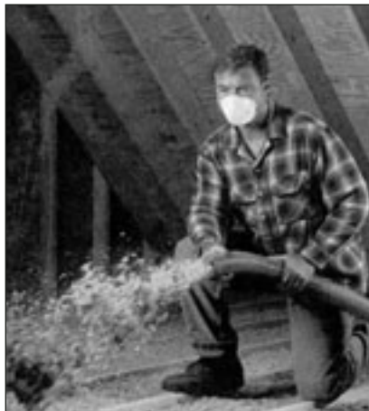
Loose-Fill Cellulose Insulation (Left), Damp-Spray Cellulose (Right).
