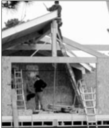
Construction using SIPs
