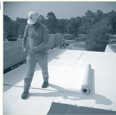
Cool roof sheathing being installed on a flat roof.
