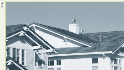
Durable roofing tiles such as these look like wood shake but will last 40 years or more.
