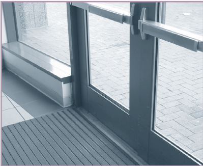
Permanent entryway grilles like this one help reduce tracked-in contaminants at central entrances.
