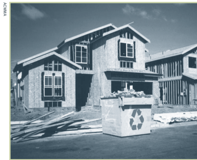
Jobsite recycling bins.
