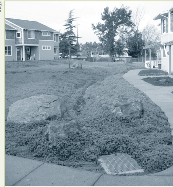
Swales are attractive landscape features that absorb and filter stormwater runoff, reducing pollution.
