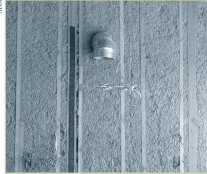
Cellulose insulation completely fills voids that would otherwise be difficult to insulate with fiberglass.
