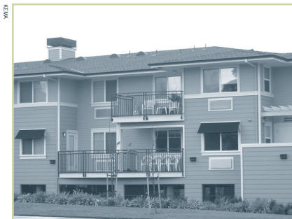
This tuck-under garage allows for natural ventilation with minimal visual impact.
