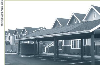
Solar panels can double as covered parking.
