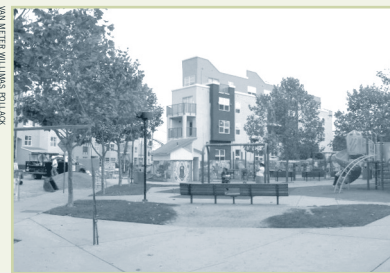
Multifamily green buildings can blend harmoniously with contemporary design. The Nueva Vista project in Santa Cruz creates inviting spaces—inside and out.
