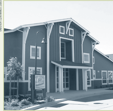
Common rooms, such as this building at Murphy Ranch in San Jose, are an integral part of multifamily living.
