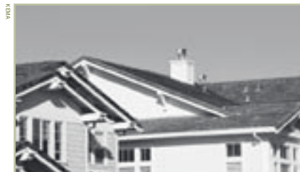
Durable roofing tiles such as these look like wood shake but will last 40 years or more.
