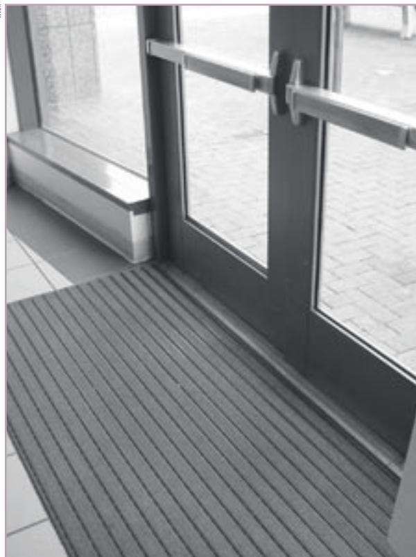
Permanent entryway grilles like this one help reduce tracked-in contaminants at central entrances.
