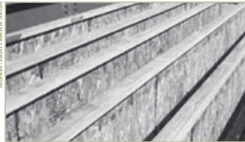
I-beam floor joists use up to 50% less wood fiber to perform the same structural function as similarly sized solid-sawn lumber.
