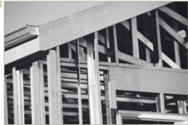
Steel-framed building detail.
