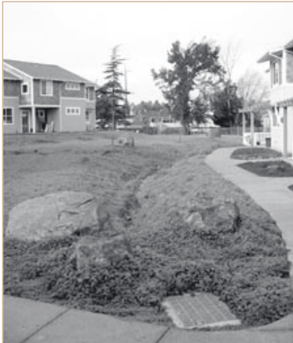
Swales are attractive landscape features that absorb and filter stormwater runoff, reducing pollution.
