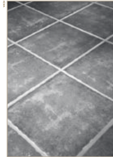
Dark colored tiles absorb and store the sun's heat in a passive solar house.
