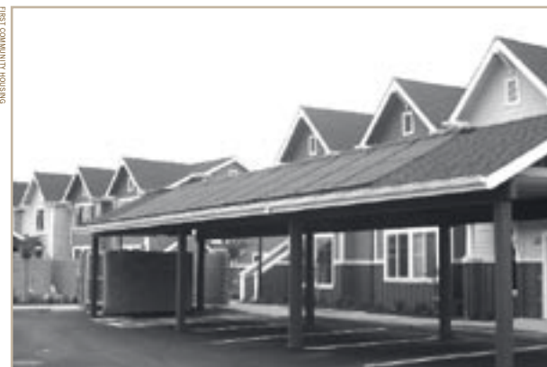
Solar panels can double as covered parking.
