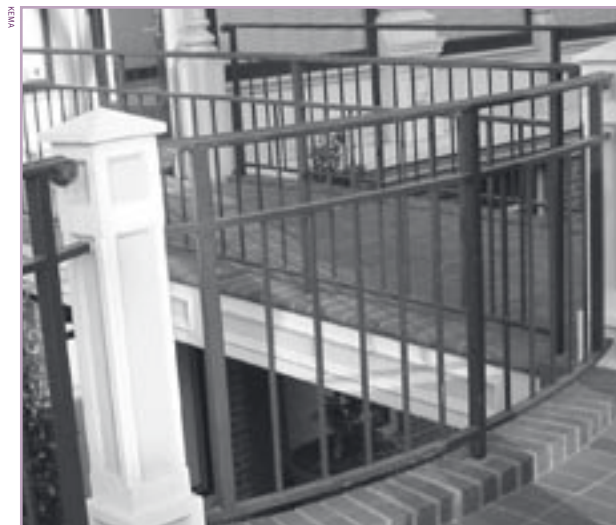
Factory-applied coatings on metal railings reduce onsite exposure to toxic materials and limit hazardous waste.
