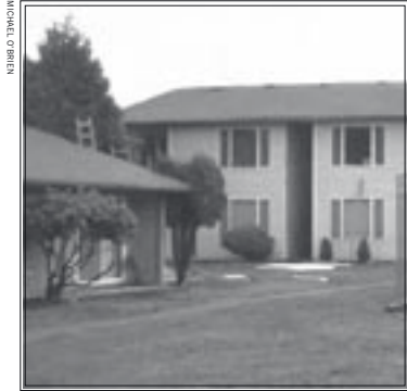
Double-pane, low-e windows were installed to increase energy efficiency.
