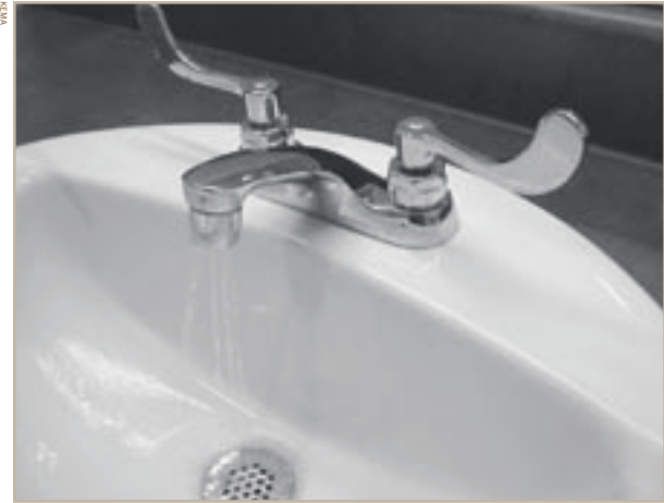
Faucets with laminar flow restrict water use.
