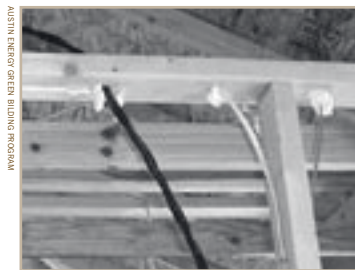
Sealing around penetrations in the building envelope reduces infiltration.
