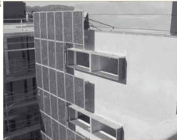
These photovoltaic panels are integrated into the building exterior at the Colorado Court affordable housing project in Santa Monica.
