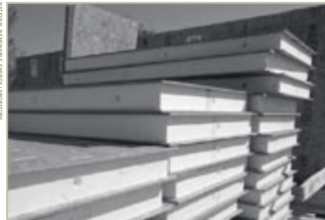
SIPs on a jobsite await installation.
