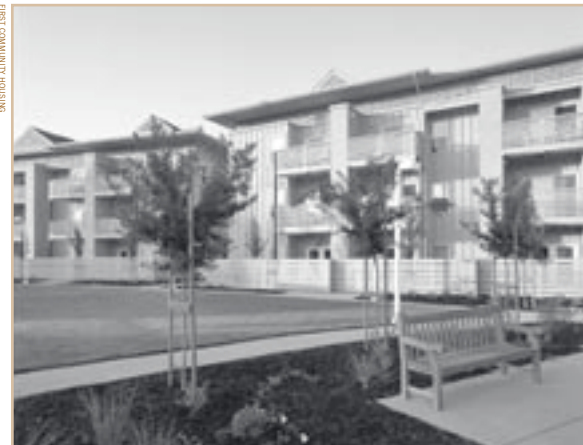
The courtyard at Betty Ann Gardens has many elements for natural surveillance: balconies that look toward a central area, benches to encourage leisure time, and proper site lighting.
