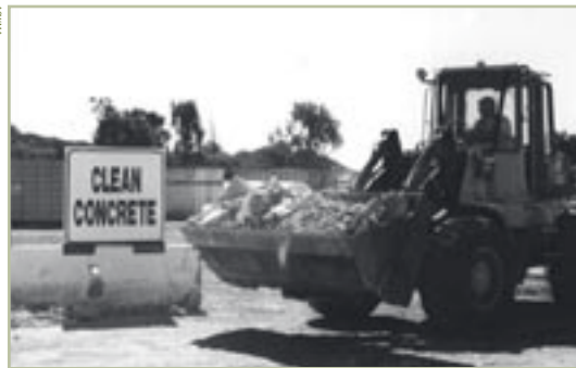
Concrete being sorted for reuse as aggregate.
