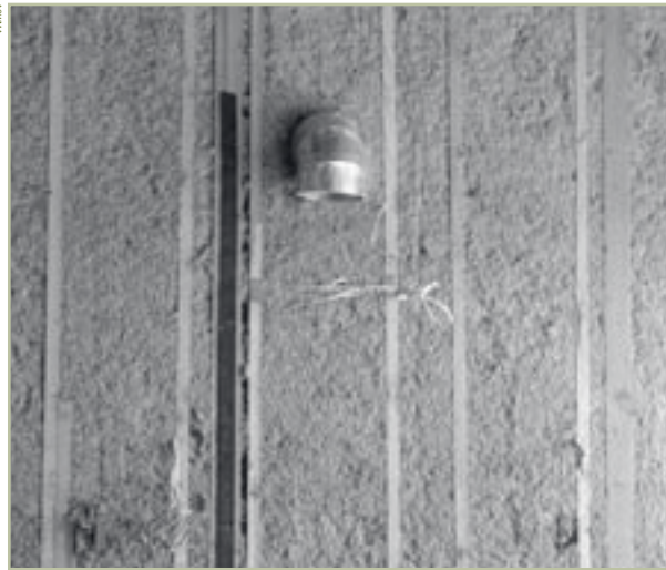
Cellulose insulation completely fills voids that would otherwise be difficult to insulate with fiberglass.
