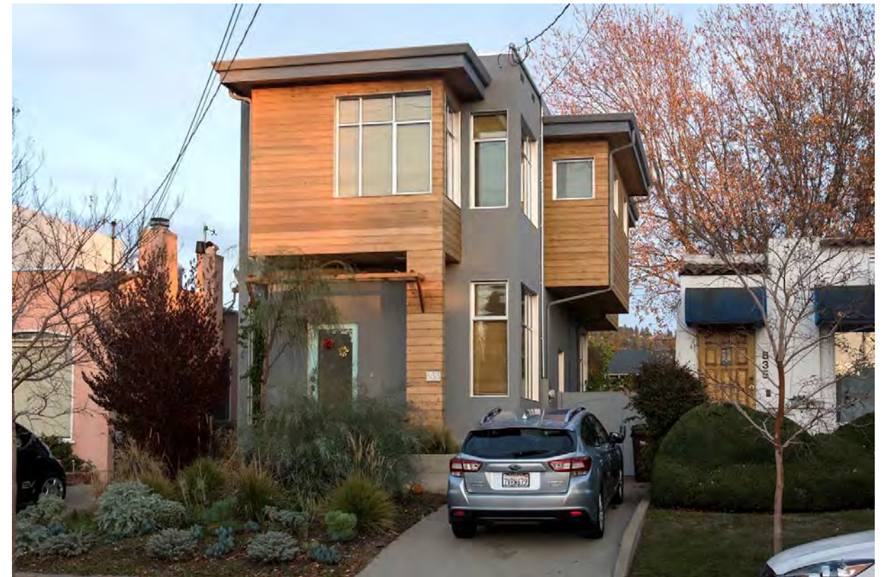
A flat roof, large window openings, horizontal slat cedar siding to accentuate projecting bays, and a modern color palette highlight the modern design.
