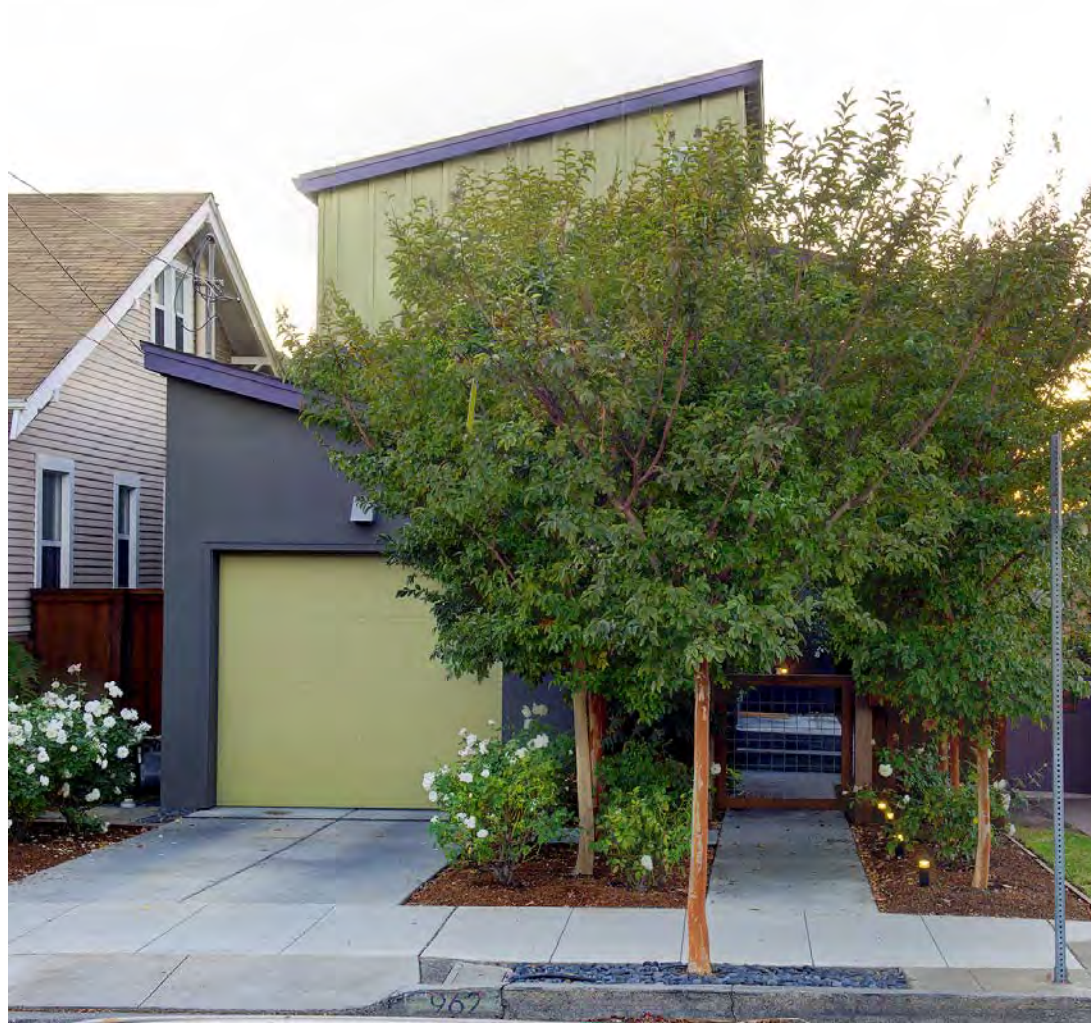
The use of shed roof, board and batten siding, and a striking color palette contribute to the modern aesthetic.
