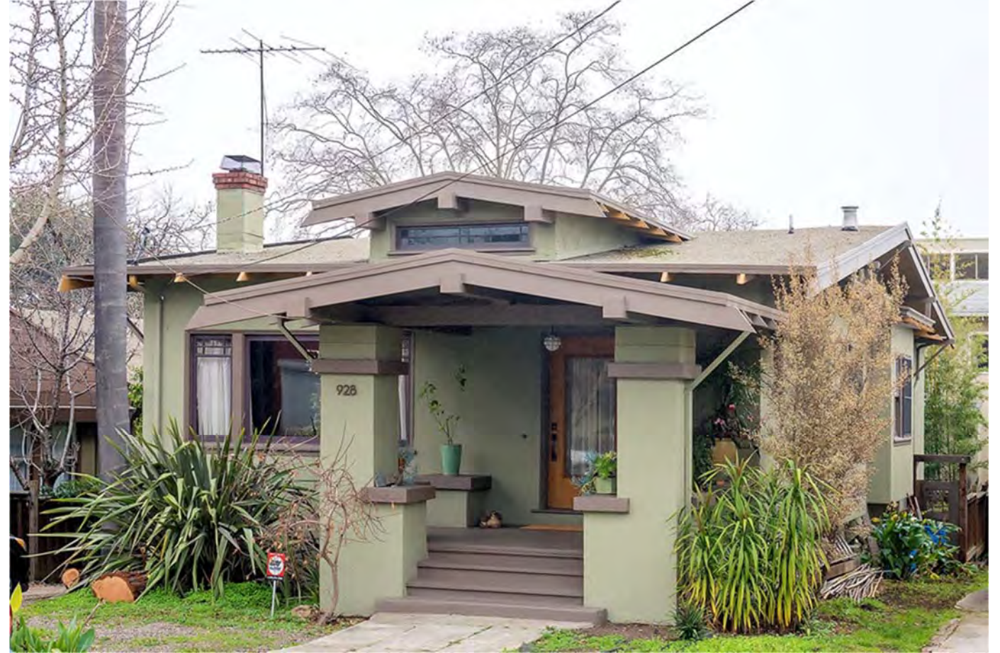
This home represents the Craftsman architectural style with decorative brackets, rafter tails, gable covered entry and cross gable roofline.
