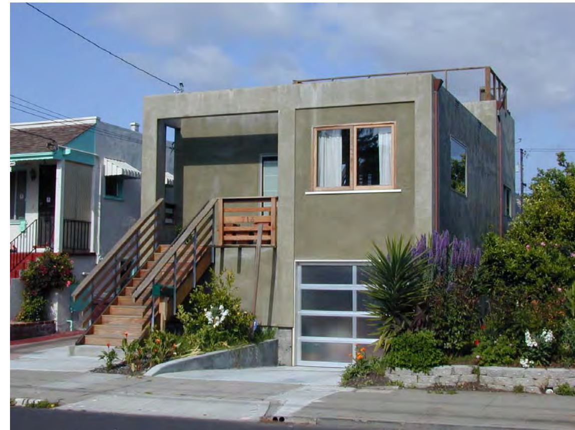
This home has a contemporary building form, modern garage door with an aluminum frame and frosted glazing, and a roof deck.
