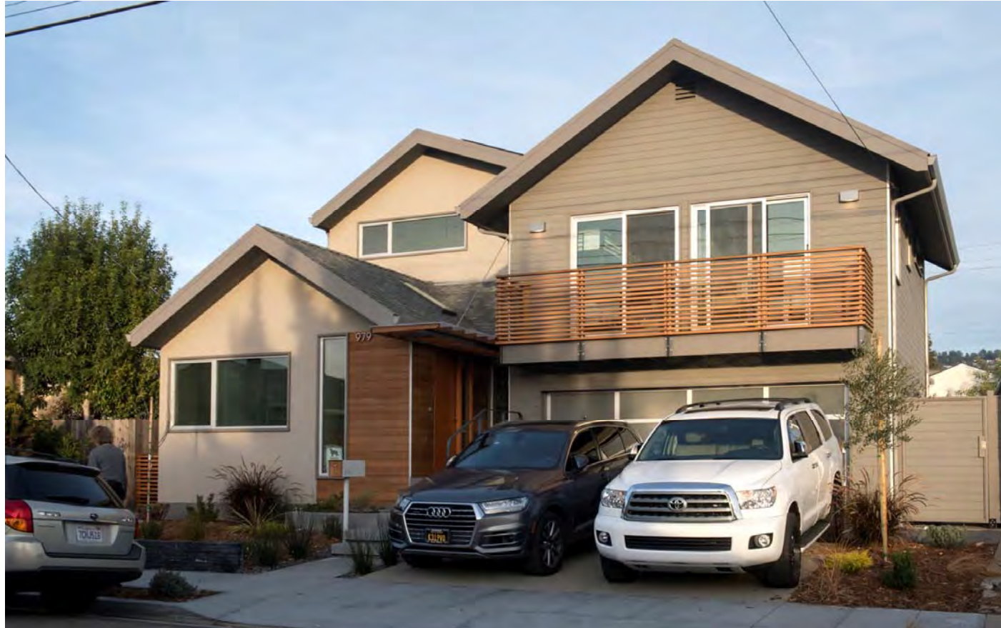
This house incorporates a blend of traditional architecture with the roof forms and contemporary details such as the horizontal wood paneling and metal garage door with frosted glass.
