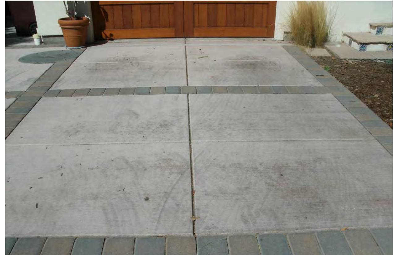
Concrete with decorative pavers
