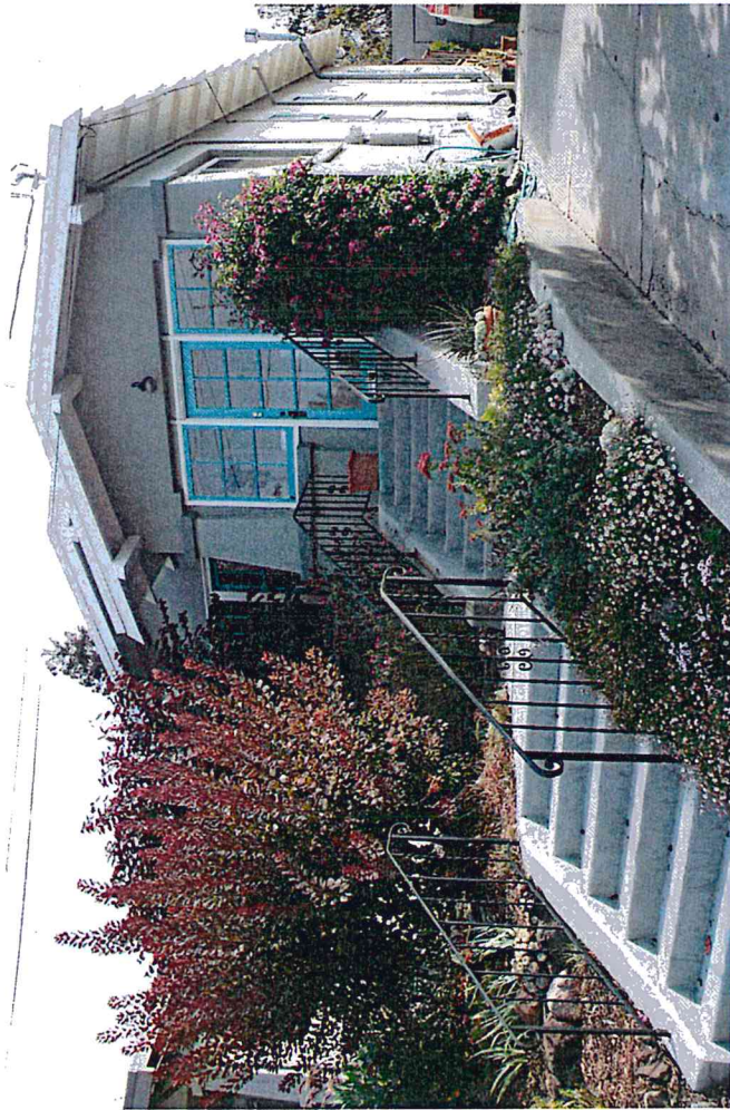
This porch is enclosed on more than two sides and counts towards the Floor Area Ratio.
