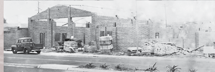
Ground breaking for the new structures was, March 17, 1965 .
