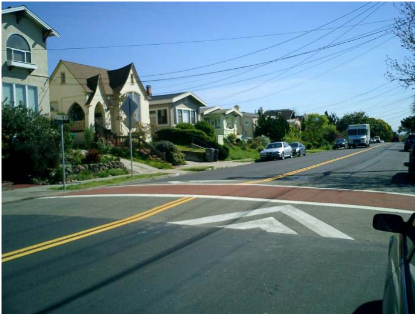
Figure 4-5 – Example of a Raised Crosswalk
