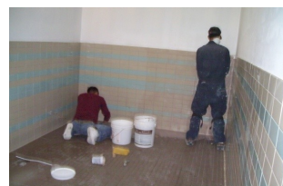
A brand-new restroom
