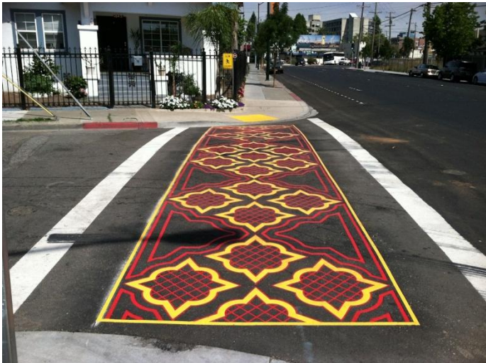
Recently installed stamped crosswalk on Foothill.
