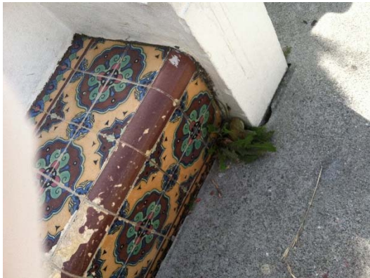
3 & 4 Close ups of deteriorating tilework of bench seat behind WW I memorial
