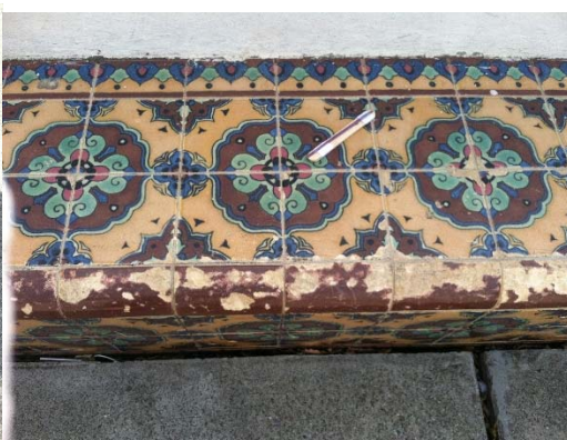
3 & 4 Close ups of deteriorating tilework of bench seat behind WW I memorial
