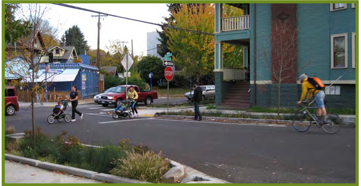
Curb extensions (bulb-outs) expand the pedestrian zone, provide space for amenities like planting and bike racks, and shorten crossing distances.
