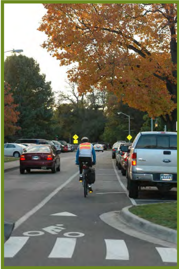
Clearly marking bike lanes help guide cyclists and identify the multimodal use of the street to slow down motor vehicles.
