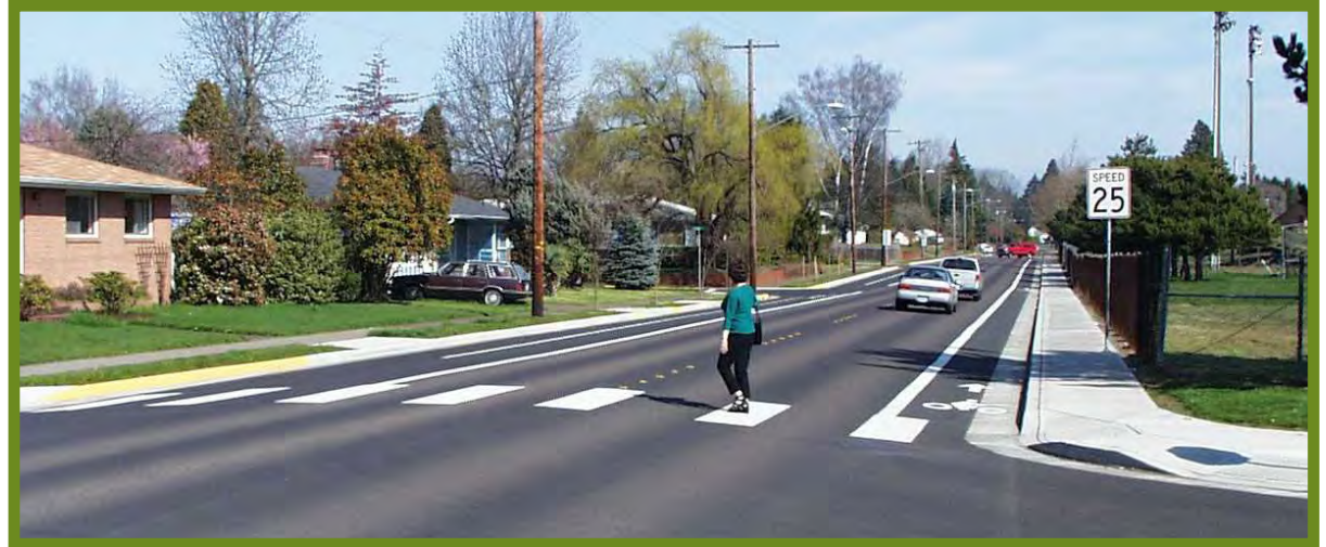
Use high-visibility longitudinal crosswalk markings for all unsignalized crosswalks. Wide lines should be spaced to avoid the wheel paths of vehicles, thus reducing maintenance costs.
