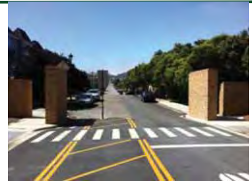
Partial closure on 15 th Avenue, north of Lake Street, San Francisco, California
