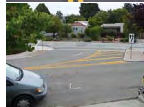
From top: Existing Santa Fe Cross Section at Solano; Sample sharrow treatment; Pomona/Santa Fe Intersection (Proposed Bicycle Turn Lane Location)
