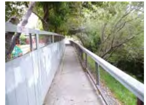
Existing portion of Cerrito Creek path
