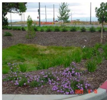
A bioretention area in Fremont provides biotreatment and some infiltration of stormwater runoff.
