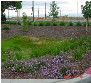
*A bioretention area in Fremont detains and infiltrates stormwater runoff.*
