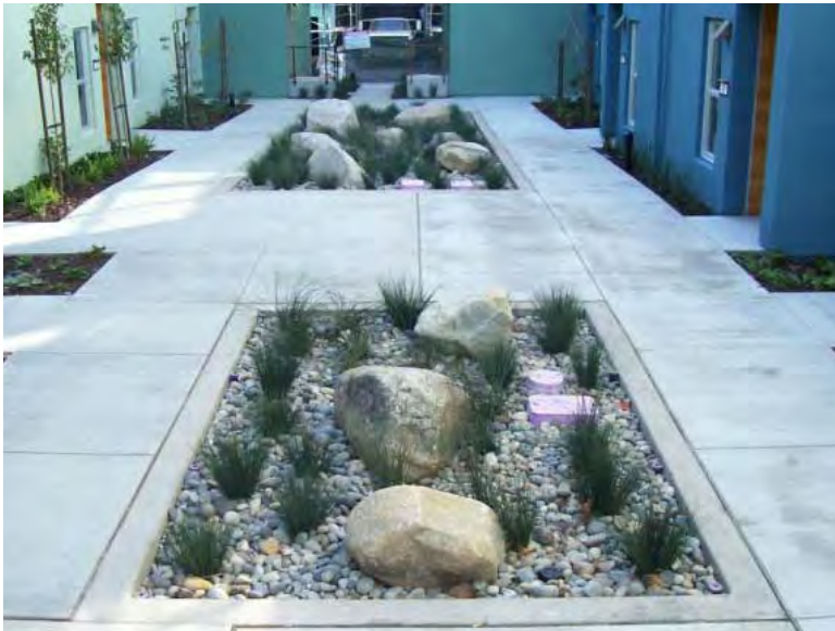
Figure 6-7: At-grade flow-through planters. Source: City of Emeryville
