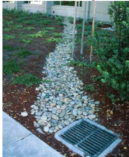
Figure 7-5: Draining roof runoff to a landscaped area is an example of hydrologic source control.
