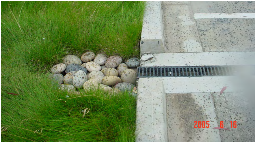
Figure 5-7: Cobbles are placed at the inlet to this stormwater treatment measure in Fremont, to help prevent erosion.
