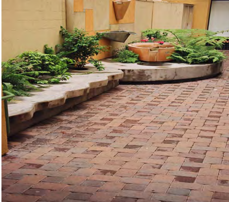
Figure 6-31: Permeable Joint Pavers at High Density Housing Project, Berkeley
