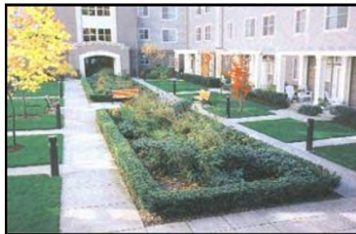
Typical Bioretention Area
