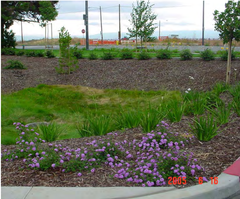
Figure 6-1: Bioretention area, Fremont
