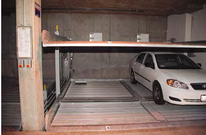
Figure 4-6: Parking Lifts in Parking Garage, Berkeley
