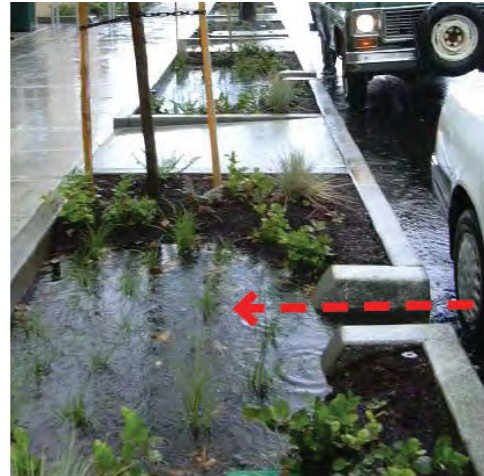
Figure 5-11: The side wings of this standard curb cut help retain the side slope grade on each side of the curb cut opening.
