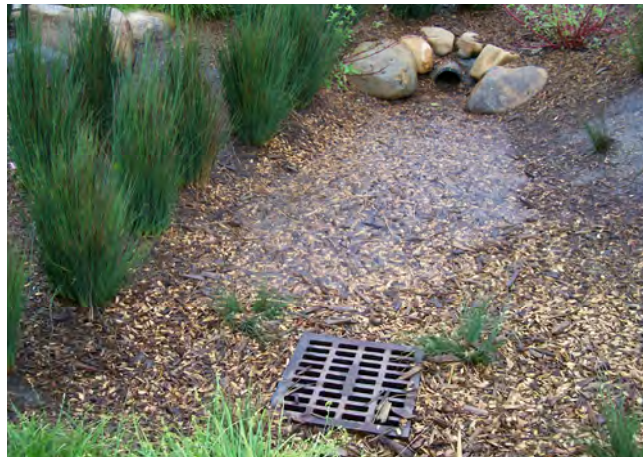
Figure 5-2: Bioretention area, Emeryville (example of a combination flow- and volume-based treatment measure)
