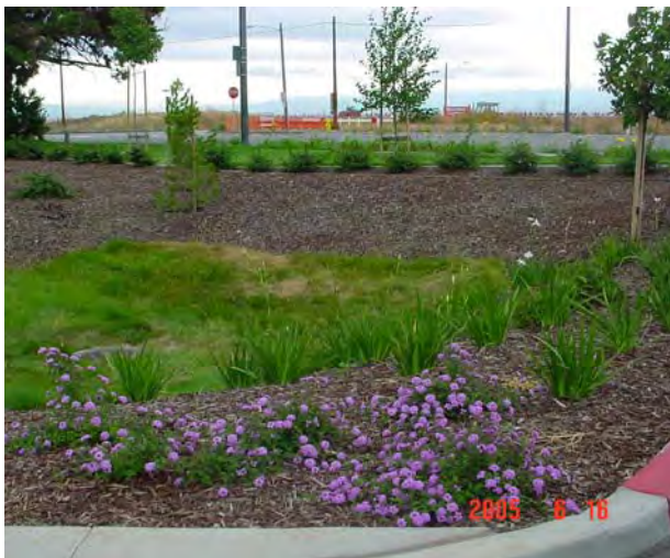
Figure 8-1: Bioretention Area in the City of Fremont
