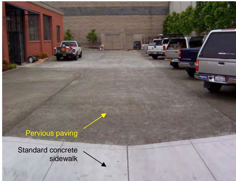
Figure 6-27: Parking Lot with Pervious Pavement, Emeryville
