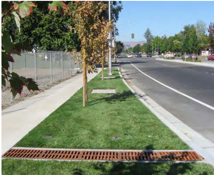
Figure 6-14: Non-proprietary tree well filters in Fremont use bio-retention soils with an infiltration rate of 5 to 10 inches per hour. Spacing the units closely together provides a total tree well filter surface area that is 4 percent of the impervious surface area from which stormwater runoff is treated.
