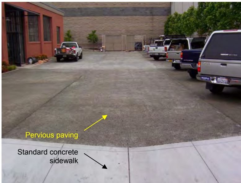
Figure 8-7: Parking Lot with Pervious Pavement, Emeryville
