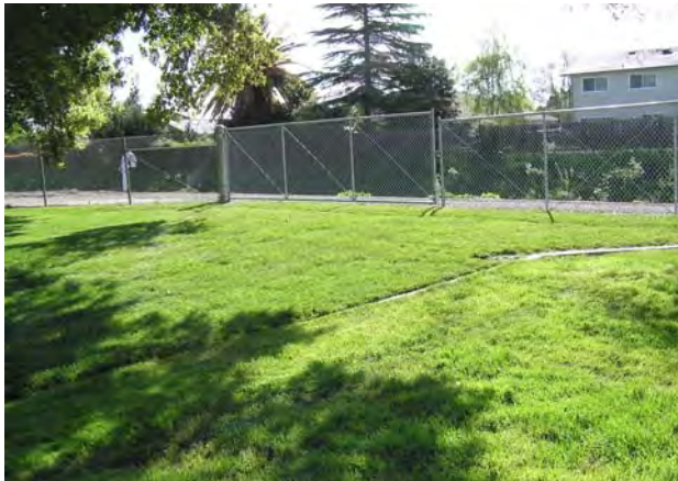
Figure 3-3: Pleasanton Sports Park includes this turf block fire access road.
