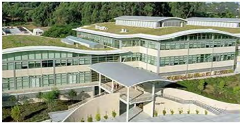
Figure 6-33: Extensive Green Roof at Gap Corporate Headquarters, San Bruno (William McDonough & Partners)
