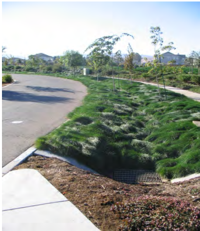
Typical Linear Bioretention Area
