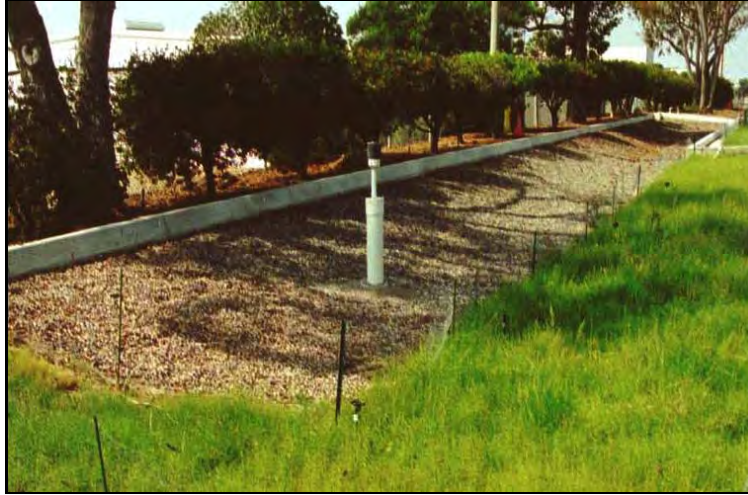
Figure 6-20: Infiltration trench. Source: CASQA, 2003
