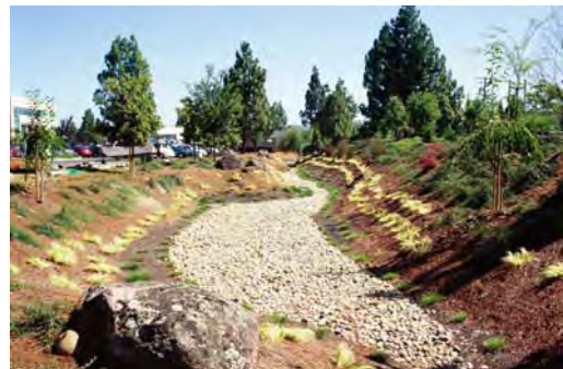
Figure 8-6: Extended Detention Basin, Palo Alto
