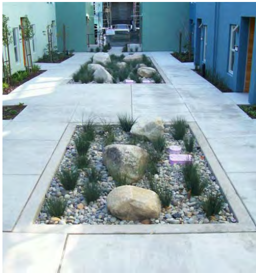
Figure 3-6: Flow-through planters are incorporated into the landscaping in a dense, urban setting in Emeryville.
