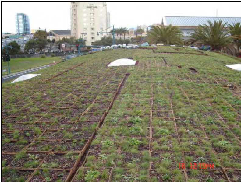
Figure 6-32: Extensive Green Roof in Emeryville
