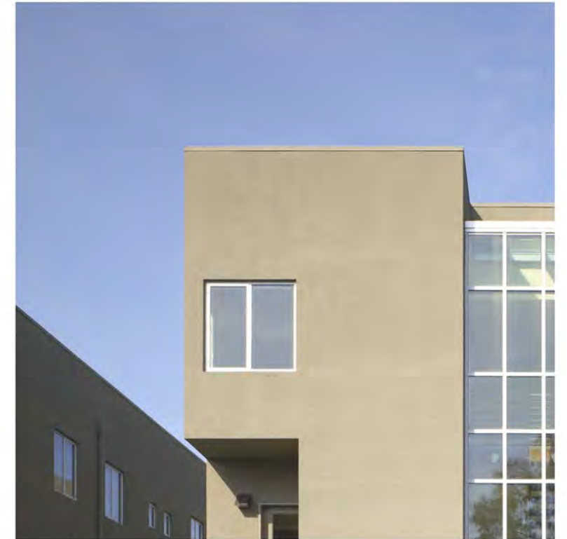
ALUMINUM WINDOWS @ CEMENT PLASTER WALL
