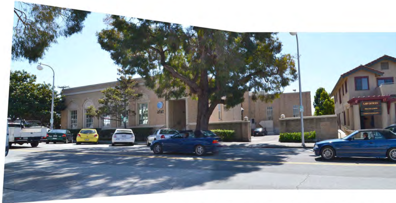
COMPOSITE PHOTO - LOOKING SOUTHEAST ON SOLANO
