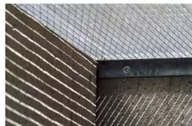
GRATE @ TRELIS WALKWAY
