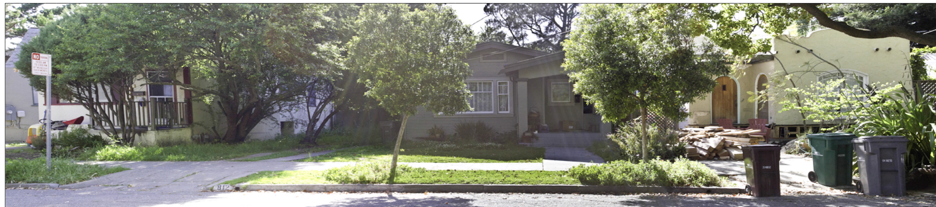
PHOTOGRAPH OF SUBJECT PROPERTY WITH ADJACENT PROPERTIES
