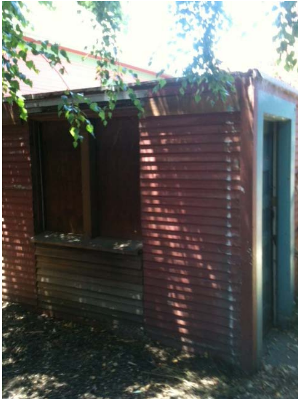
Photo 2. Rear of the Garage
