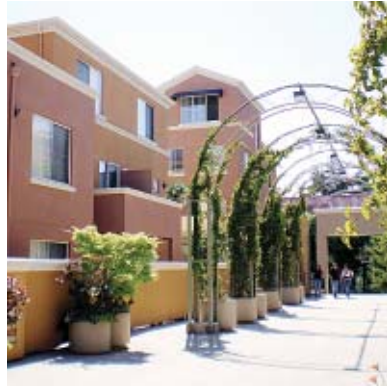
City Center Plaza, Redwood City
