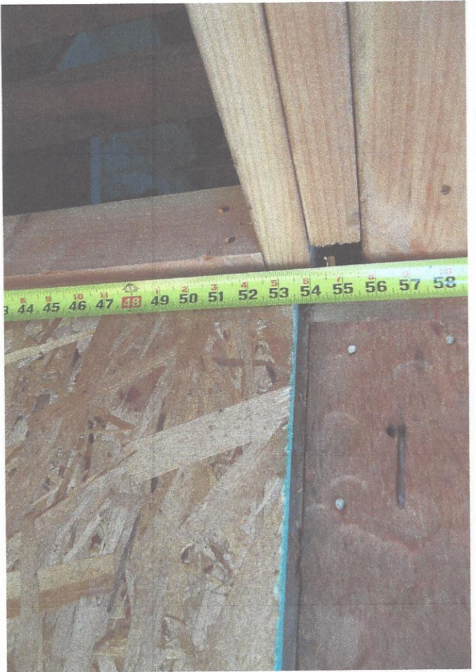
NE corner of Garage 4'6"
