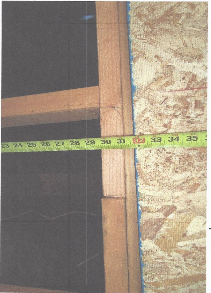
SE Corner of Utility Room - 2'8"
