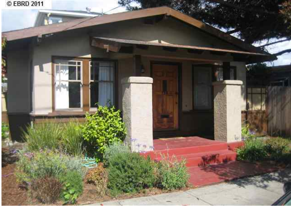
Picture 1. Stairs before work commenced
