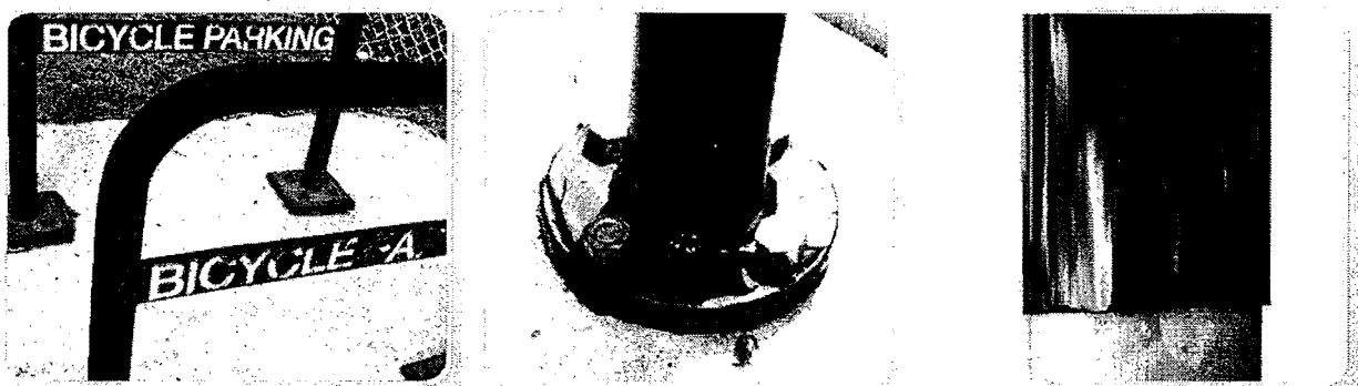
Figure 2-4: Vinyl (PVC) jacket (photos: Andrew J. Besold; John Ciccarelli; Dero Bike Racks)
