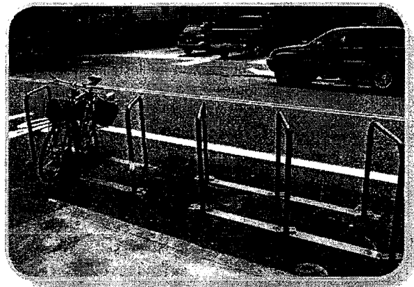
Figure 2-36: Inverted U racks are welded in clusters of three onto steel tracks in order to affix to an asphalt surface (photo: Jonathan Maus, BicyclePortland.org)
