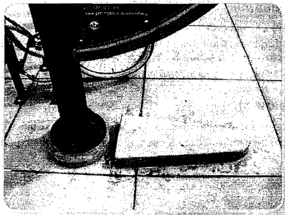
Figure 2-18: Detectable footing around bicycle parking area (photo: Eric Anderson)
