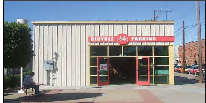
Bicycle Station at 4 th & King Caltrain Station, San Francisco
