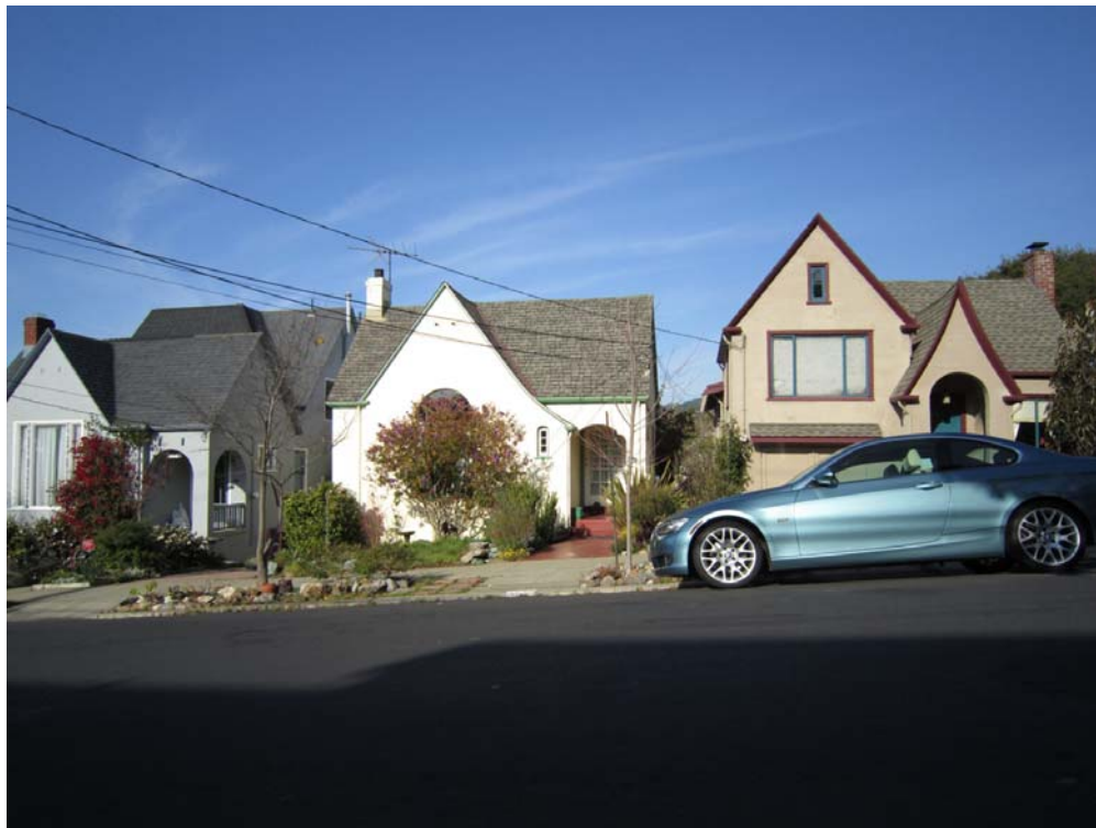
Photo 3. Neighboring homes east of the subject site
