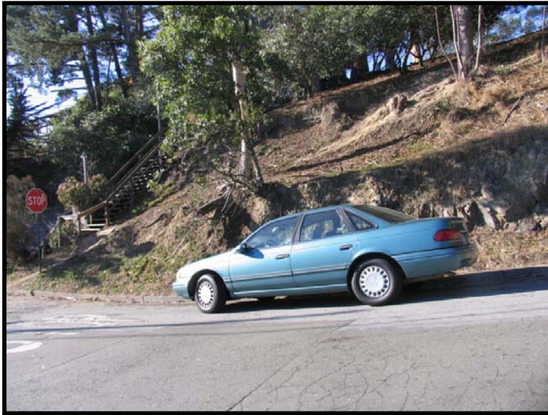
Steps at lower Taft on private property. New steps are being proposed on City owned property just north (or to the right of the privately owned steps.) #2 from the Access and Circulation recommendations.
