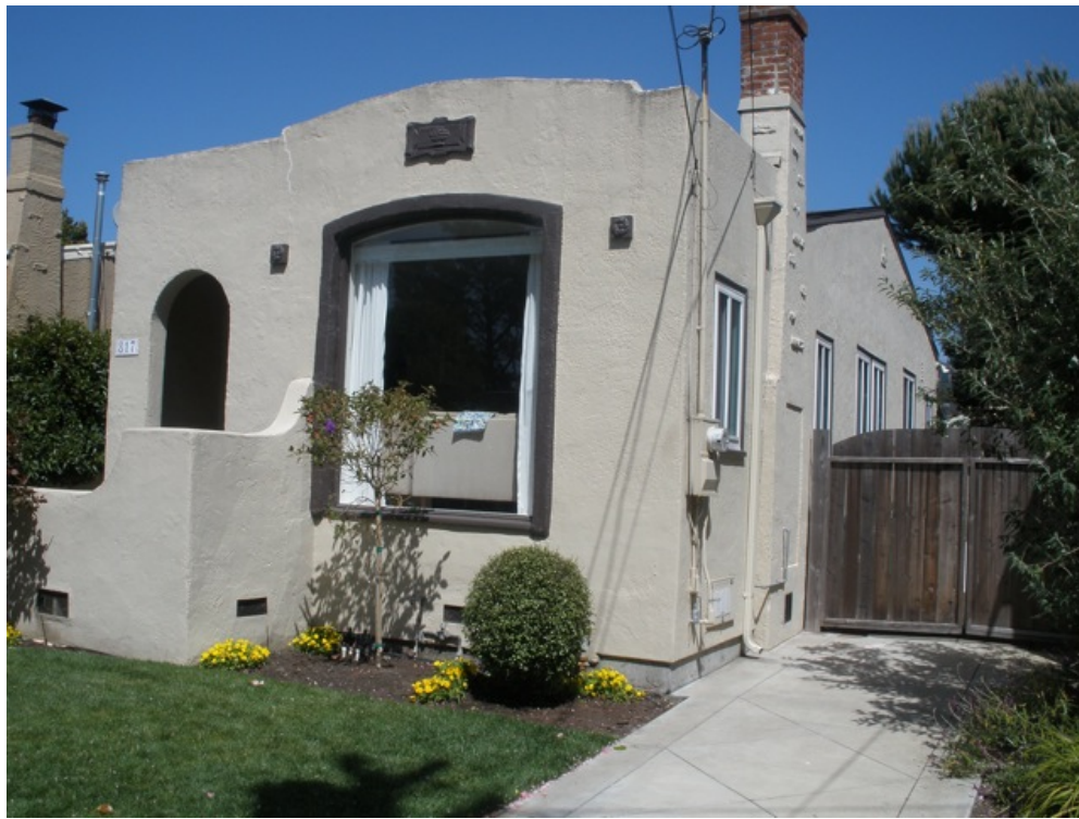
Photo 1. Street View of the existing home
