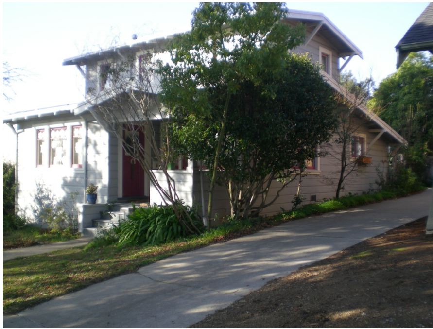
Photo 4. North side of the home
