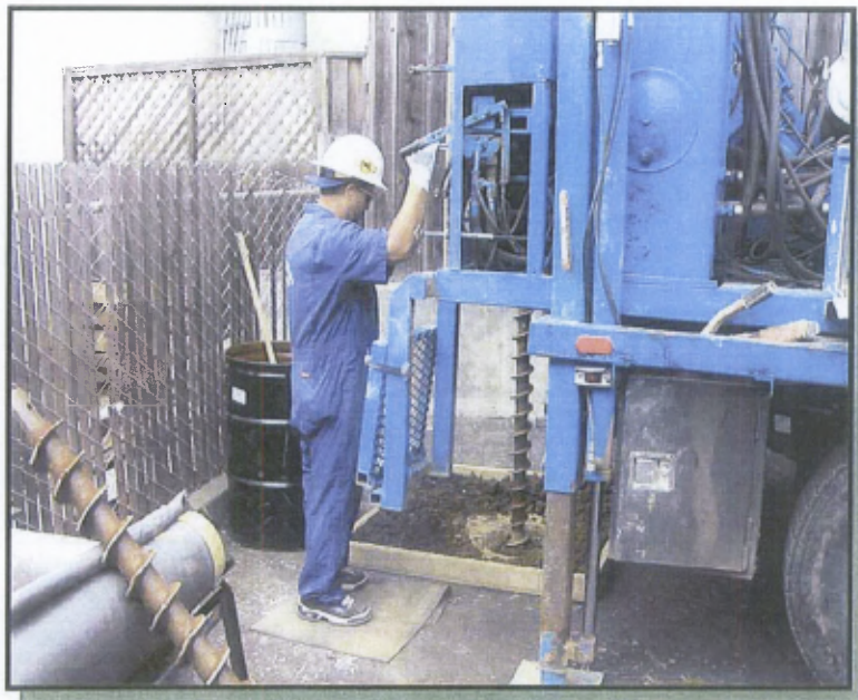
Photograph of Drilling Operation
