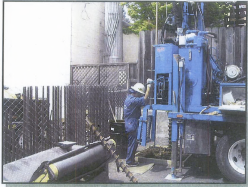
Photograph of Hollow Stem Auger
