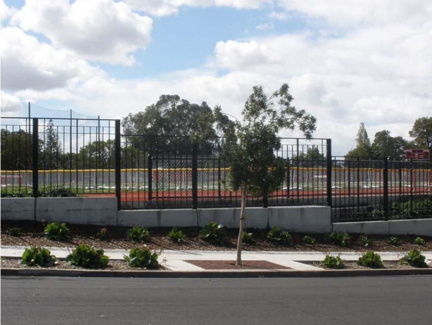
Image 44 – St. Mary's street walls along Posen Avenues
