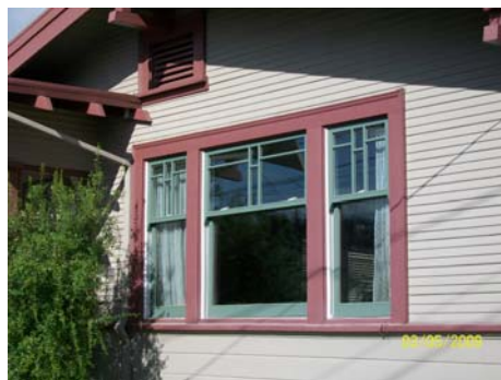
2" window recess from face of wall
