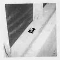
**Bolts** secure your home's mud sill to the concrete foundation. The mud sill should be bolted at four to six-foot intervals (as specified on your prescriptive plan set).
