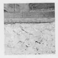
Faulty materials such as rotten wood and porous concrete should be replaced. Risky conditions in concrete include cracks wider than 1/8 inch, large volds, or "honeycomb" concrete. If the concrete chips or flakes when you poke it with a screwdriver. it may be unsafe. NOTE: If you suspect faulty material, you may need the assistance of a licensed engineer or architect to design a solution.
