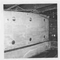
Sheets of plywood nailed to the cripple walls help to prevent damage from shaking in this typically weak area of your house. Cross-bracing within the framing is not enough.
