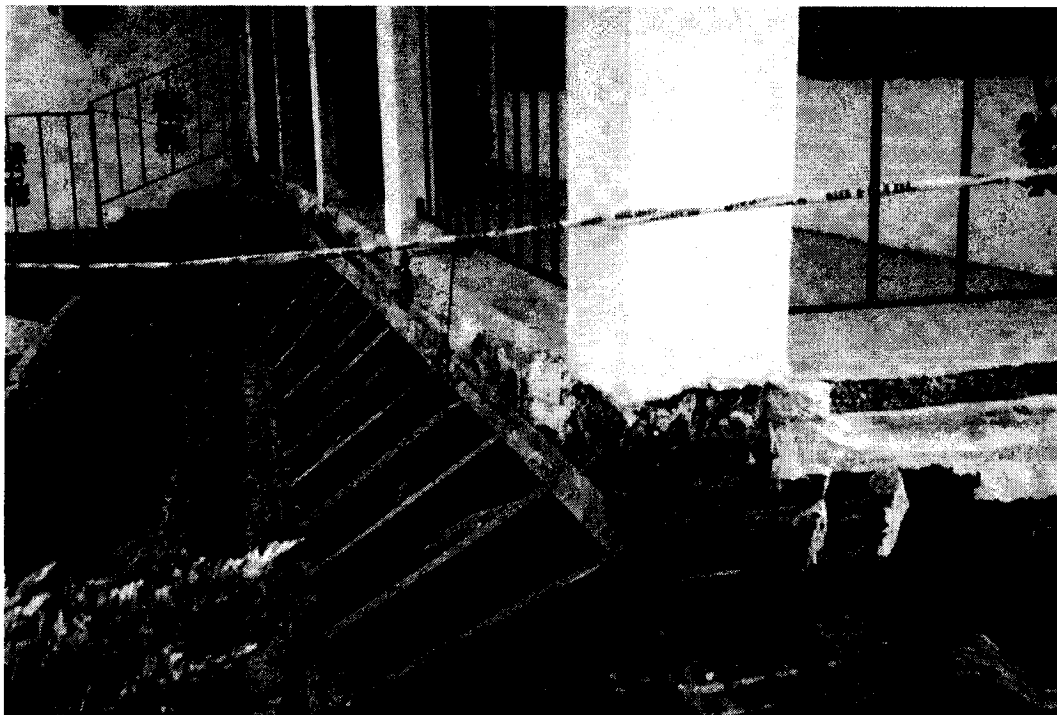
Figure 5. Cripple wall damage in the Northridge earthquake
