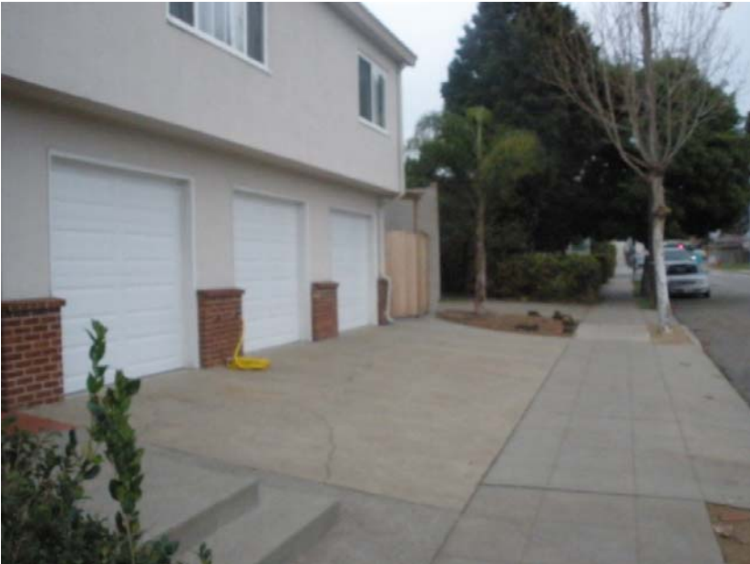
Image 33 –Apartment garages – doors/ façade opportunity here
