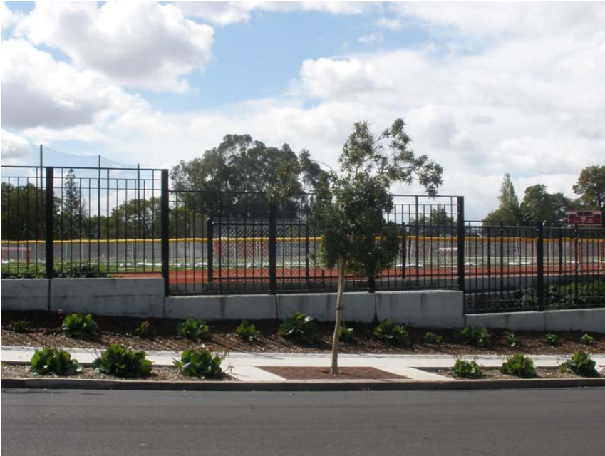
Image 44 – St. Mary's street walls along Posen Avenues
